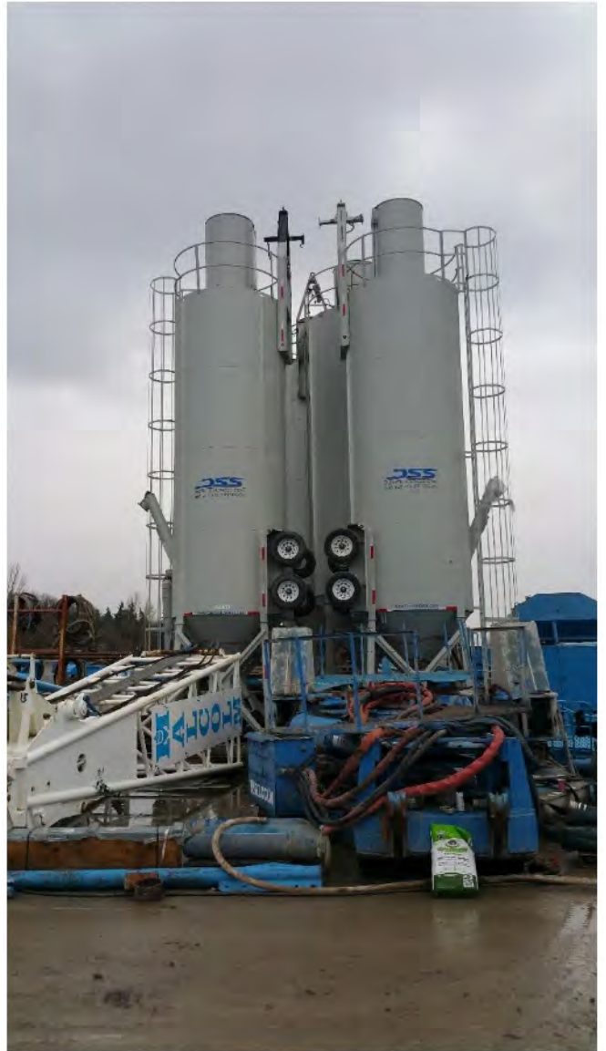
Outside Storage of Grout Silo and Equipment Components Kent, WA
