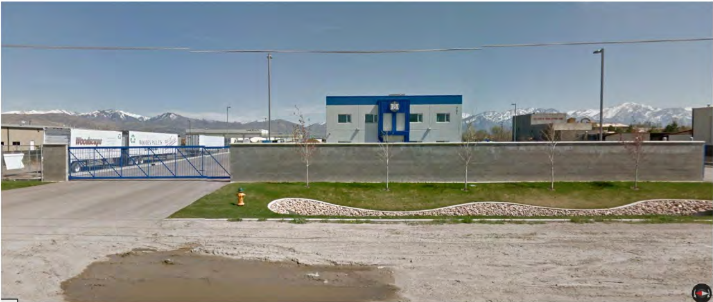
Google Street View of Malcolm Facility in Salt Lake City, UT
