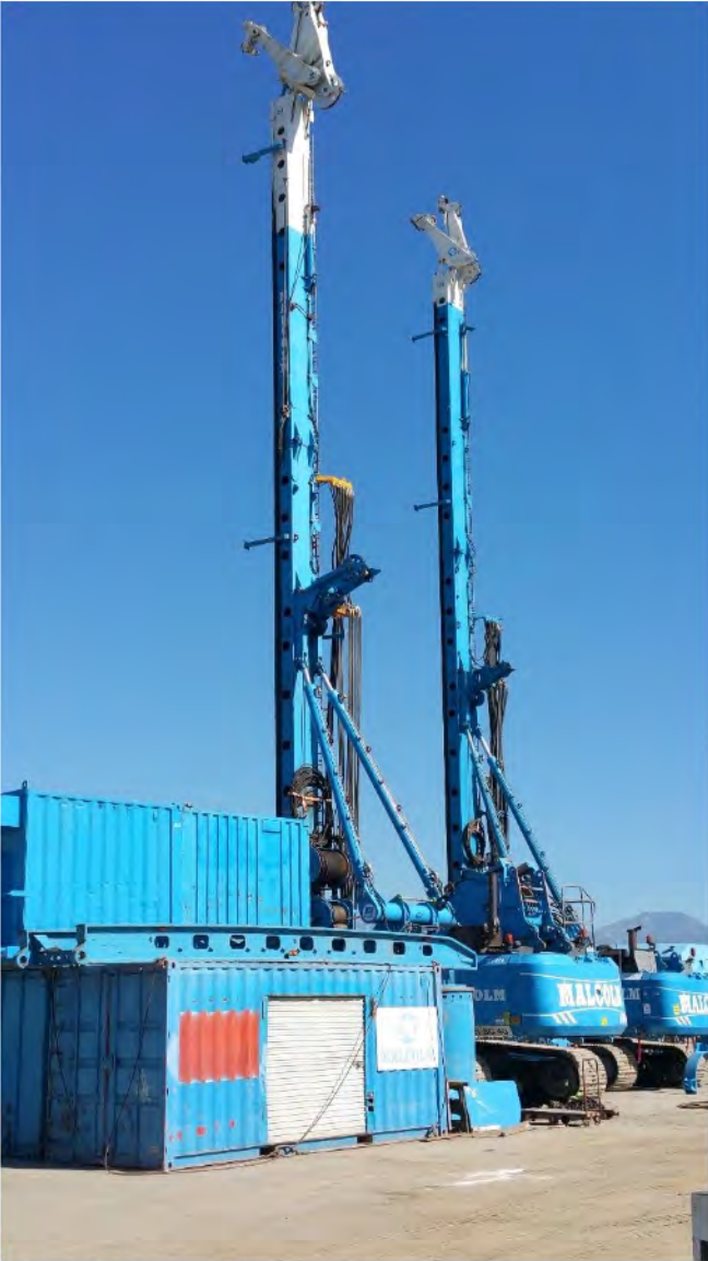
Outside Storage of Drilling Equipment and Shipping Containers - Hayward, CA
