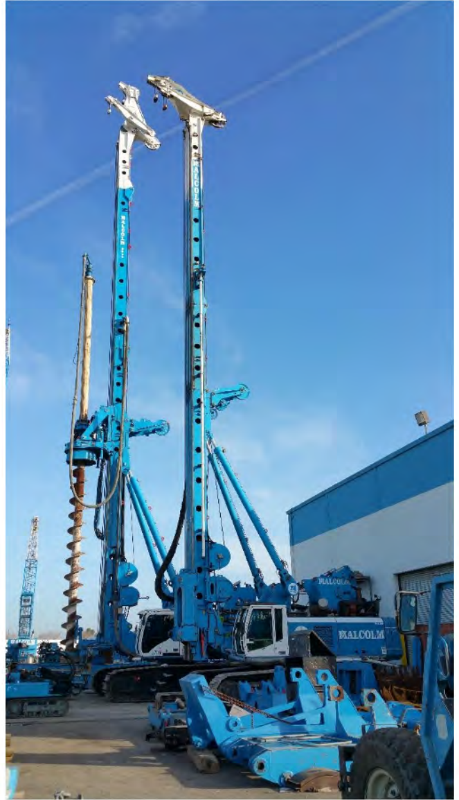
Outside Storage of Drilling Equipment - Hayward, CA
