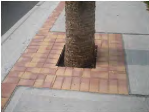
Trees are planted within either grass or brick paver terraces. At major and minor intersection types, the Paver Grate system shown above should be used as opposed to an exposed steel tree grate.
